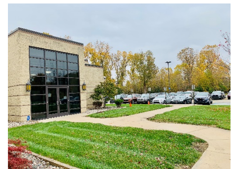
Major repairs to the Church building's roof and subsequent leak damage were accomplished by the trustees in 2020.
